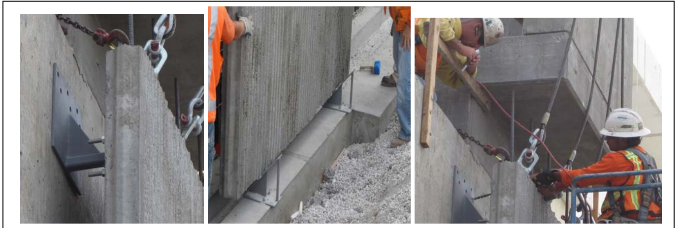
Figure 18: Modified Connection at Side Abutment Locations
