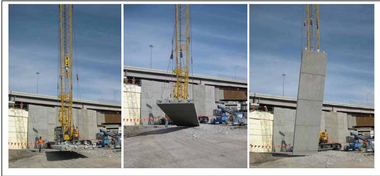
Figure 15: Rotation to Install Precast Wall Panel
