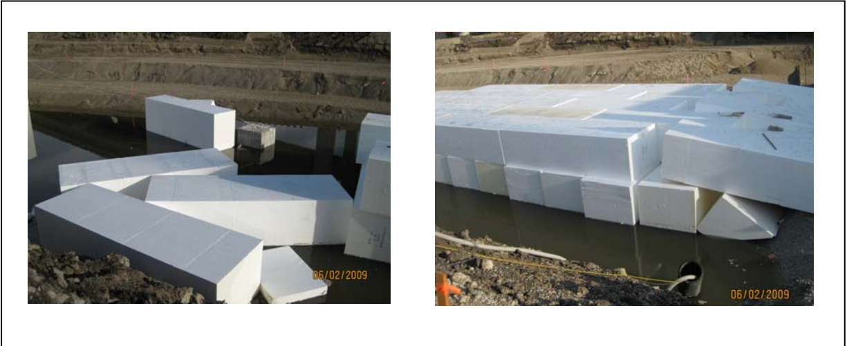
Figure 22: Buoyant Geofoam after Groundwater Level Raised
