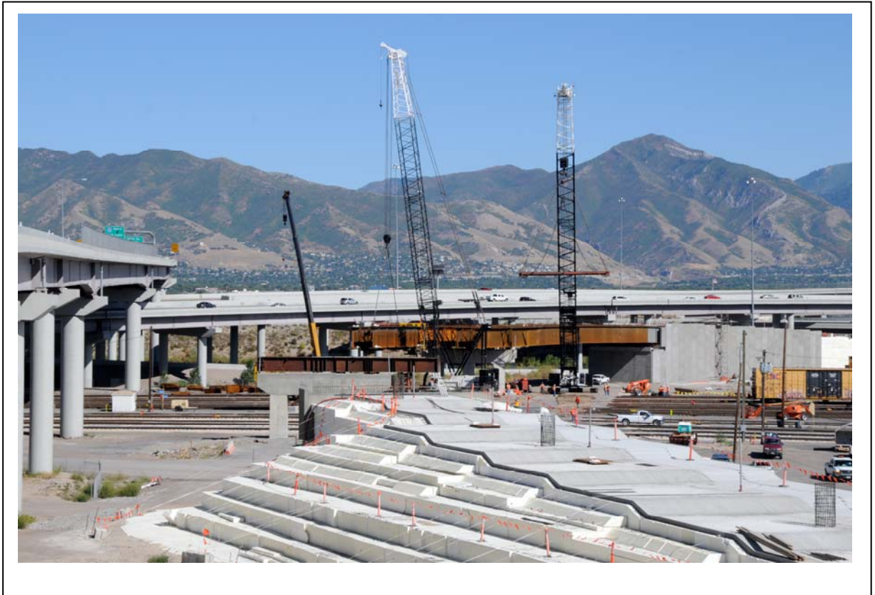
Figure 11: Load Distribution Slab Steps
