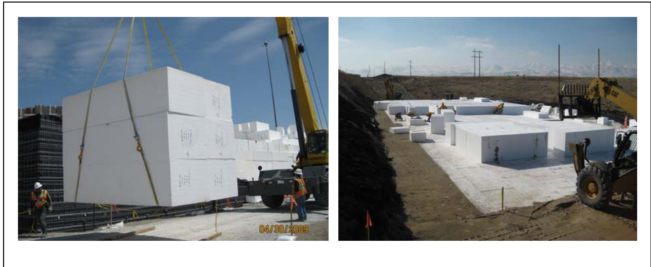
Figure 7: Geofoam Placement
