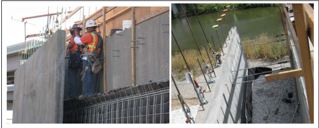
Figure 17: Tilt-Up Panel Connection at Abutments
