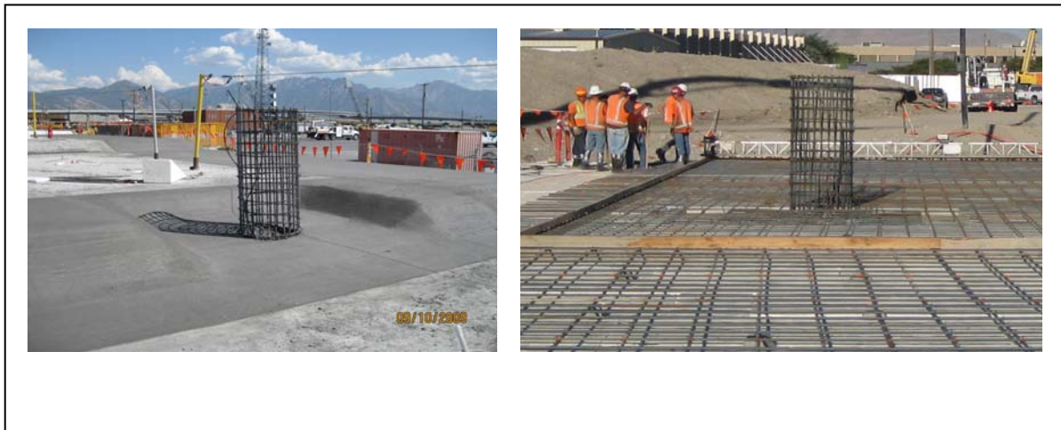
Figure 21: OCS Foundation in Load Distribution Slab
