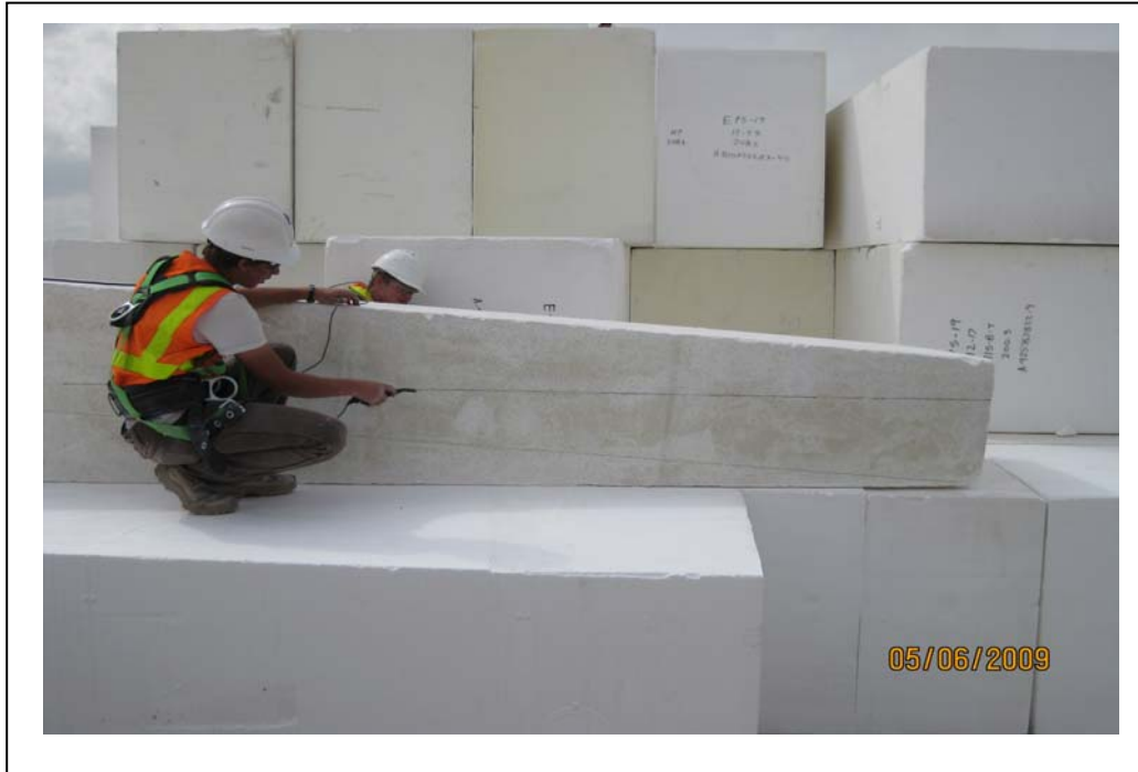
Figure 10: Cutting Geofoam
